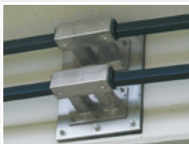
▲ Duct fixings for bridge tensioning constructions
