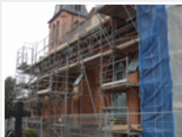
▲ Groß Escherde church: Tension anchorages with bricked-in end plates
