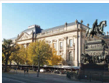
▲ National Library Berlin: Support profiles as special constructions made of Lean Duplex stainless steel
