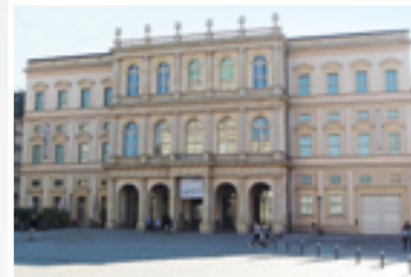
▲ Museum Barberini Potsdam: Cantilever beams made of Lean Duplex steel, 1.4062 and 1.4162
