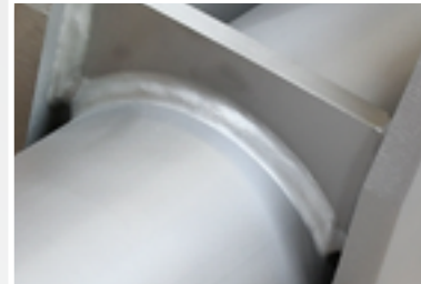
▲ Weld seam according to execution class EXC3
