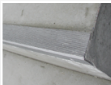
▲ Stair step protection angle - Top view
