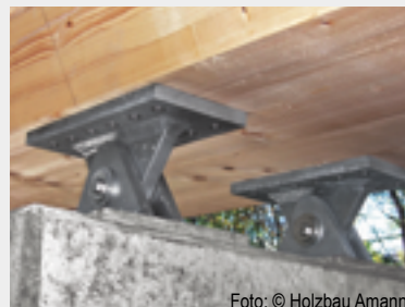
▲ Pedestrian bridge Freiburg-Ebnet: Welded constructions for supports and cut-to-size parts as custom-made products
