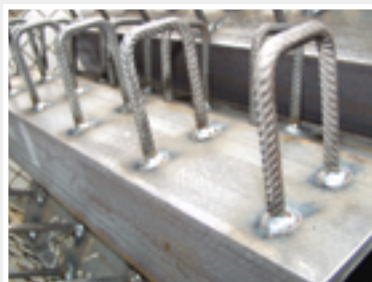
▲ Mounting bracket with reinforcing bar brackets
