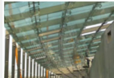
▲ Tunnel Petuelring Munich: Cable ducts with access ladders
