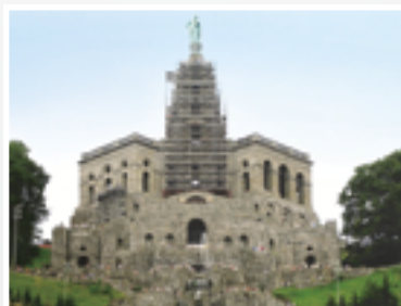
▲ Herkules, Bergpark Kassel-Wilhelmshöhe: Supports (foundation ring), reinforcements and figure supporting structures
