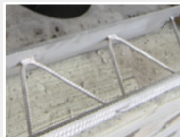
▲ Concrete reinforcement brackets
