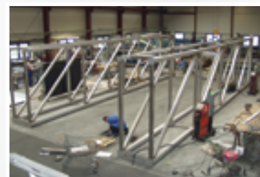
▲ Substructure North Bridge Minden
