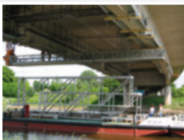
▲ Substructure North Bridge Minden
