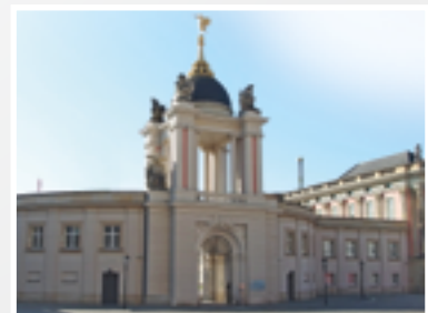
▲ Brandenburg Parliament Potsdam: Column anchors, support anchors for sandstones, cornice brackets
