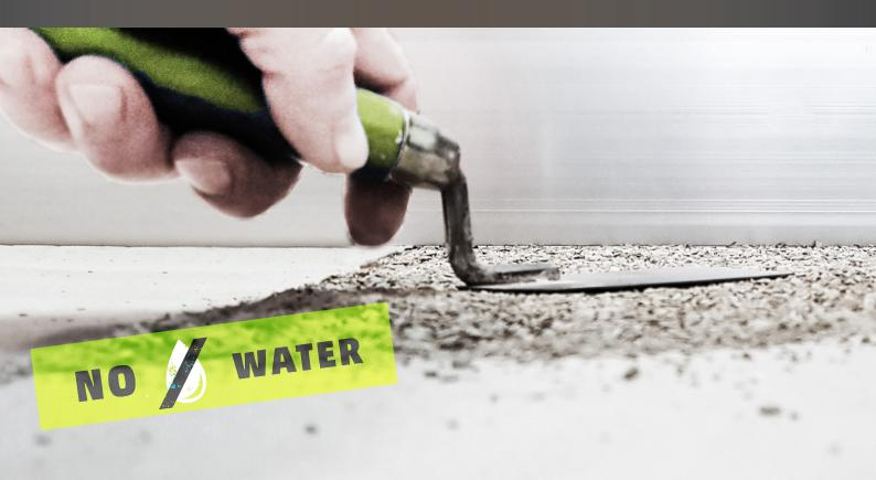
**1.** ] Dry levelling fill for small level irregularities on solid ceilings
