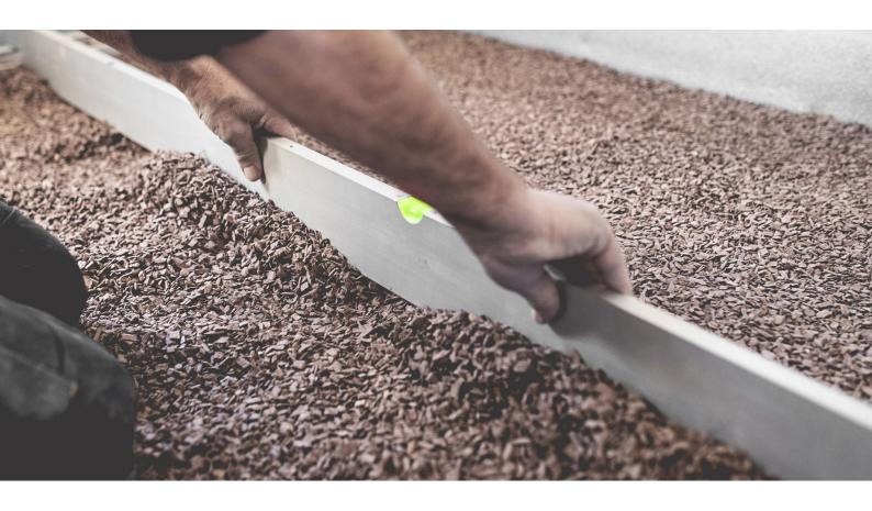
1.] Dry construction system with panel heating: on wooden beam or solid ceilings
