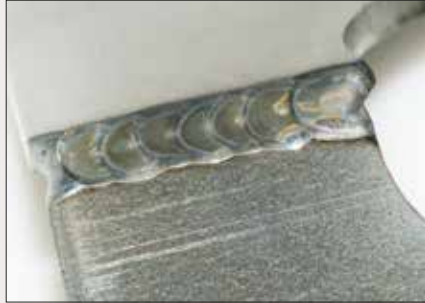
Welded joints of different materials
